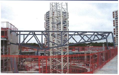
Large steel trusses are currently being installed by ISG Jackson to form Canada Water Library's roof structure. The image shows one of the larger span sections that has now been bolted into position off the main lift core (to the left of the photograph). The tower crane will perform 32 individual lifts to transport all the structural steel sections onto the roof over the course of the next two weeks.
